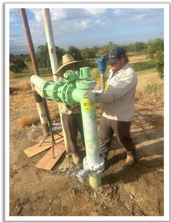
Replaced a Butterfly Valve and Air Vent at Turnout E-16
