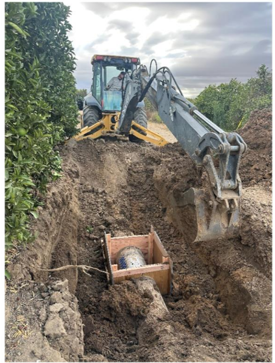
Repaired Pipeline Near Pump Plant N1-P8 Due to Leaks
