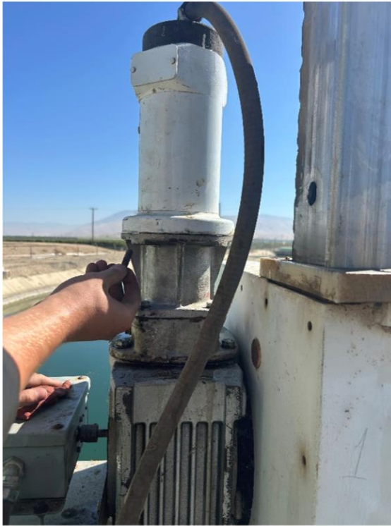
Replaced Gearbox at Check Gate 615 After Failure
