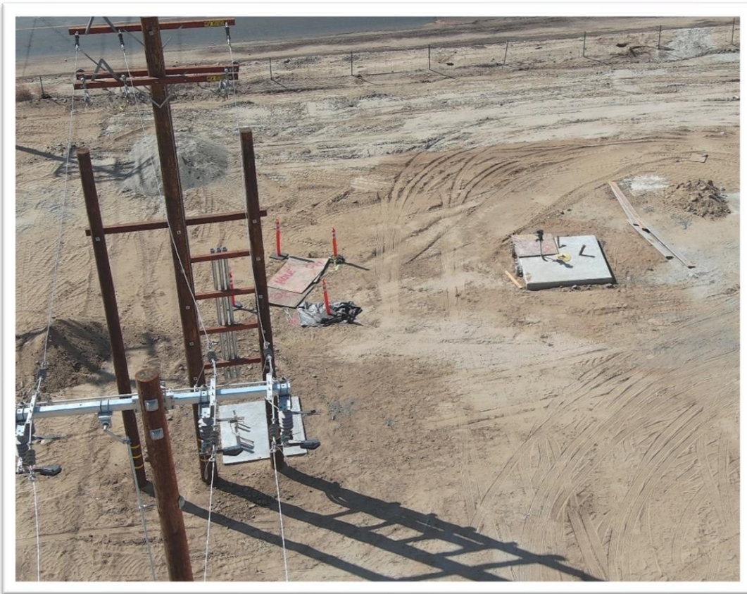
Progress of Well N26 Project Construction
