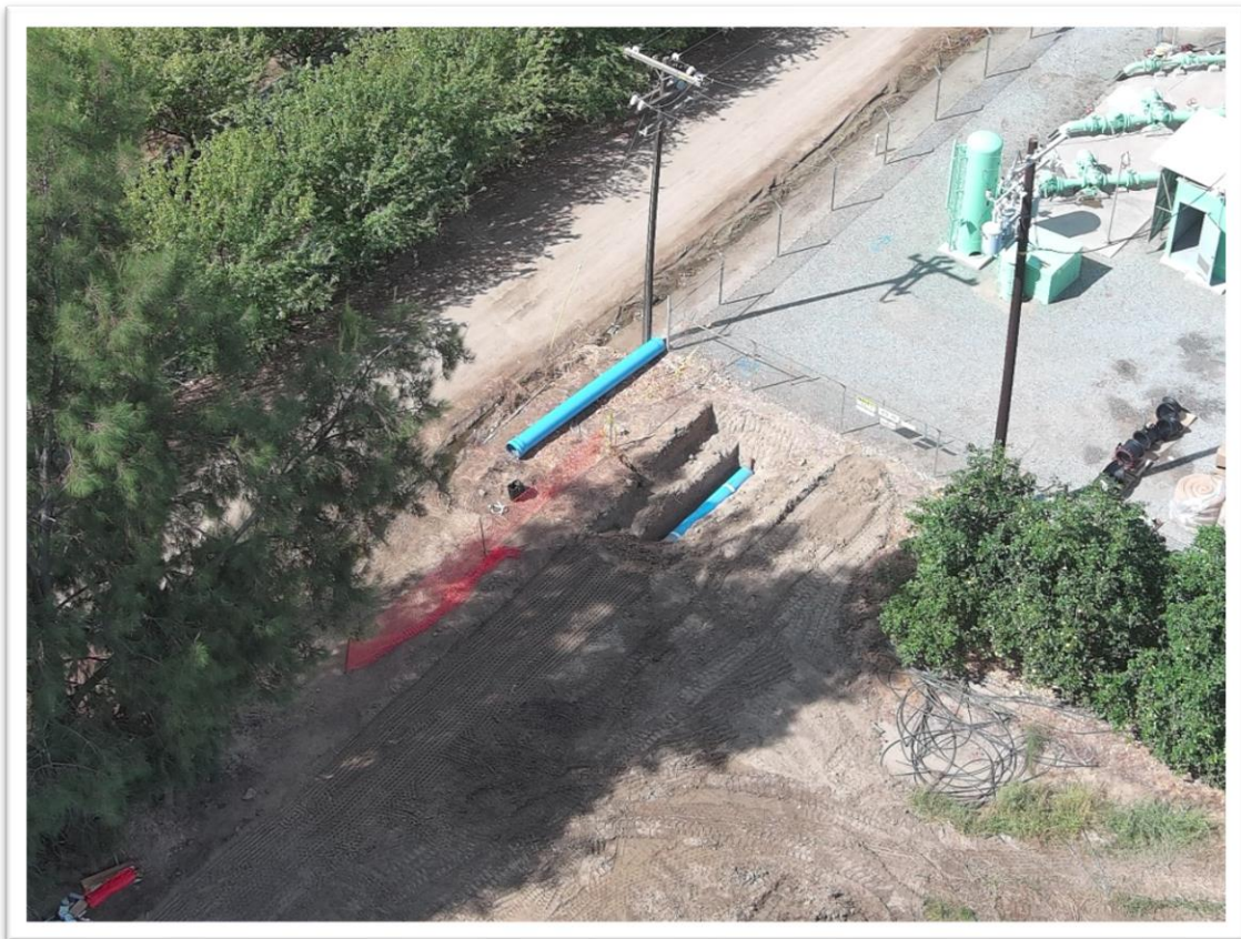
Began Construction of the 850 Canal Intertie Project
