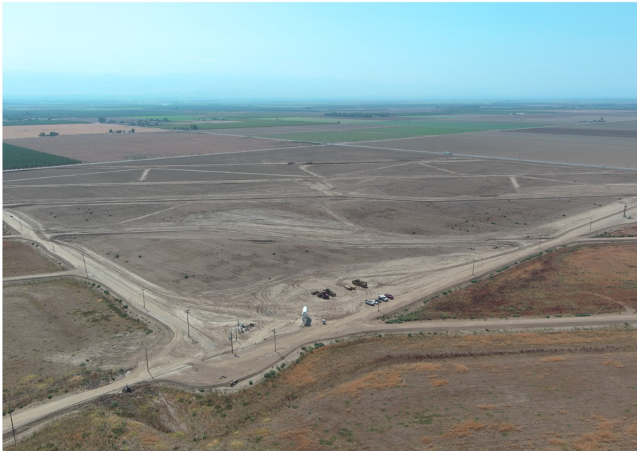
Progress of Construction of North Canal Spreading Works Expansion Project
