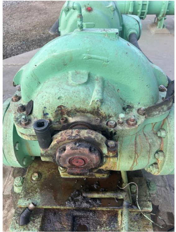
Replaced Rotating Element and Outside Bearing at Pump Plant N1-P2 Unit #6
