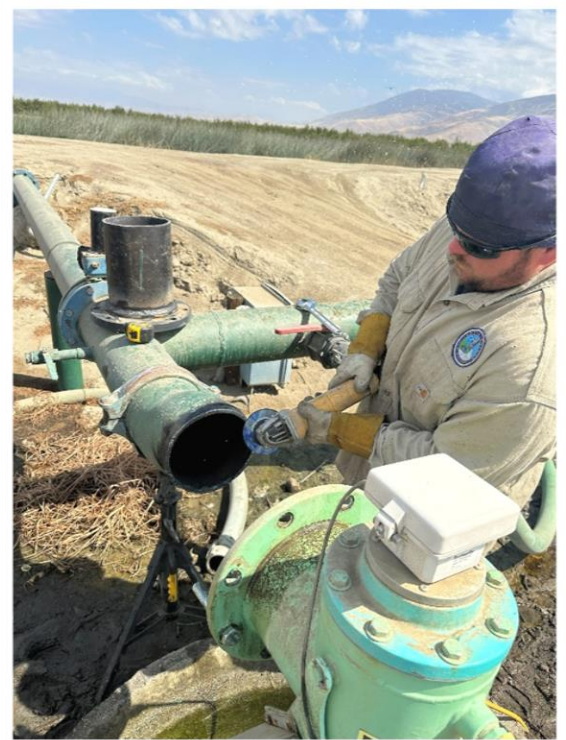
Replaced a Valve at Turnout T-83
