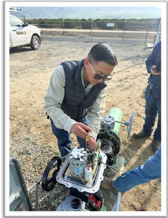
Installing a Valve at S32-P1.
