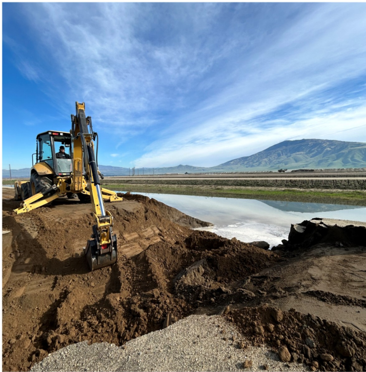
Backfilling the Blowout at Sycamore Spreading Works Row 6 Pond 4.
