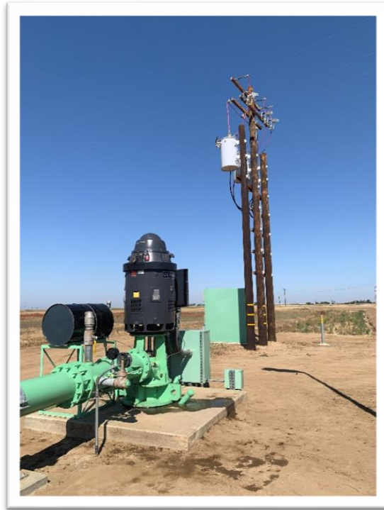
Oversaw N24 and N26 Well Startups
