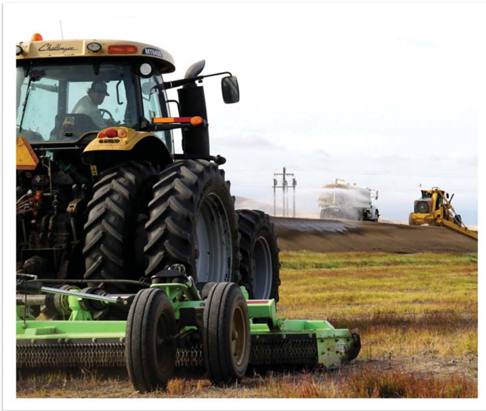
Site Clean-Up, Grading, and Mowing at Sycamore Spreading Works
