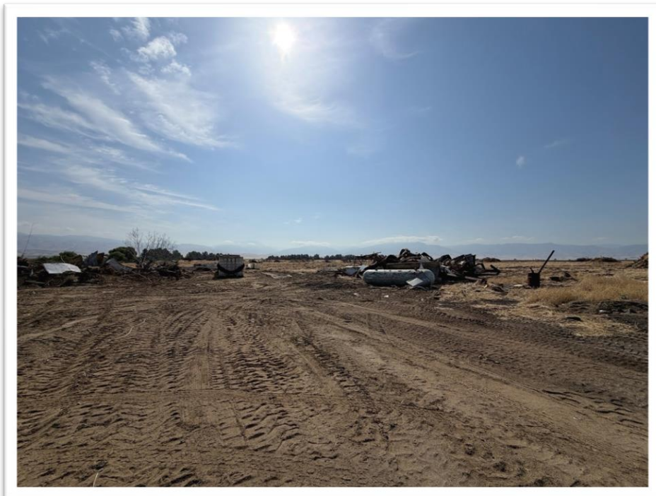
Debris Removal at El Paso Property
