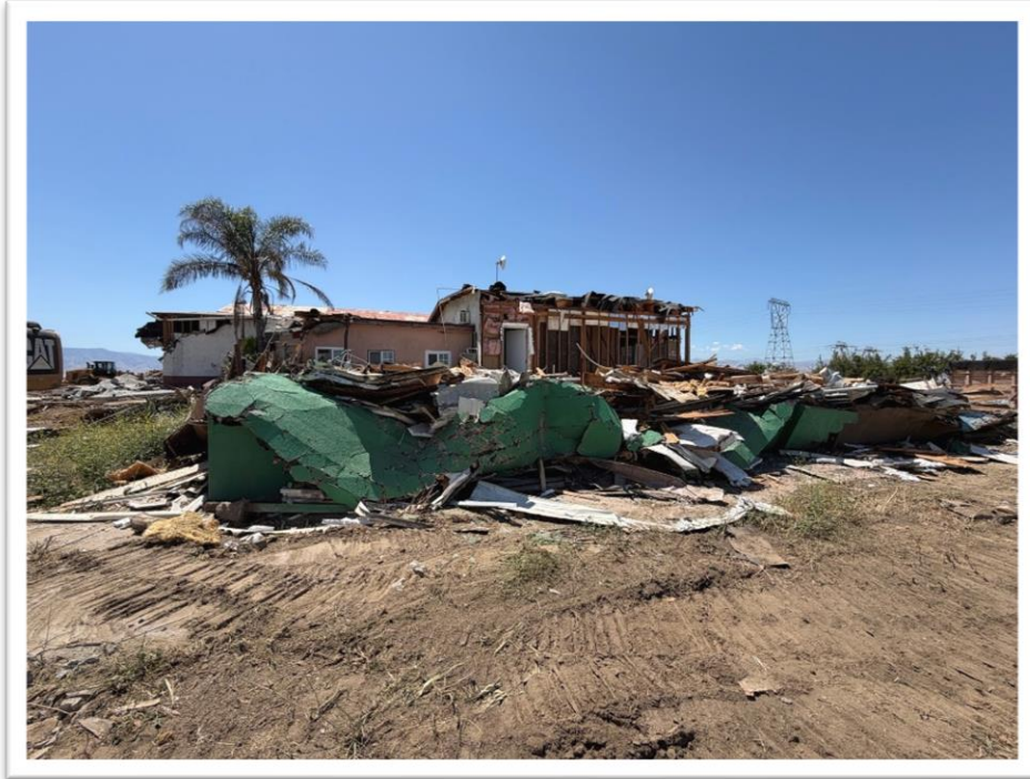
Building Demolition and Debris Removal at El Paso Property
