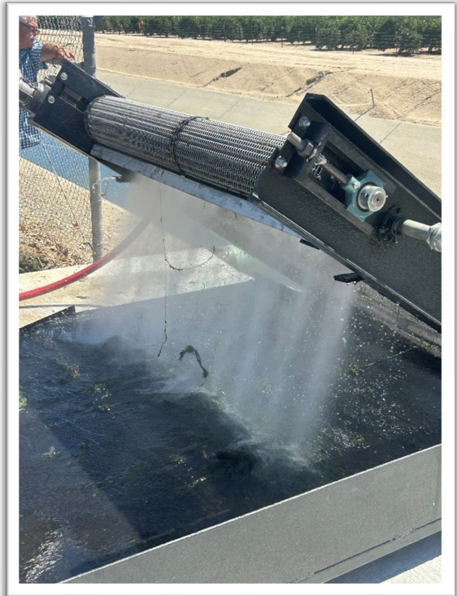
New Moss Screen Installation at Pump Plant S32-P1
