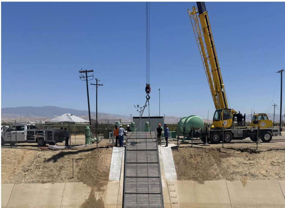
Installing Moss Screen at Pump Plant N8-P1
