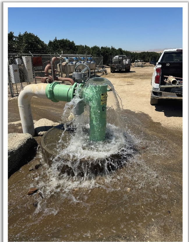
Flushing Turnout C-17
