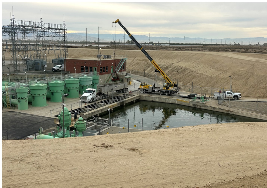
Forrest Frick Pumping Plant Forebay Seven (7) Sediment Clean-up
