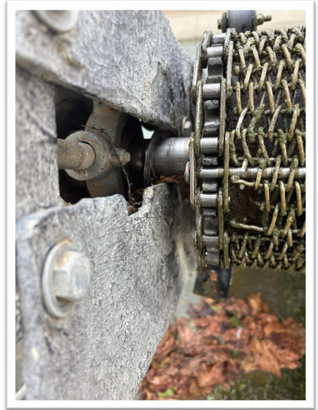
Repaired Moss Screen at Pump Plant S73-P1 Due to Bad Bearings and Alignment Issues
