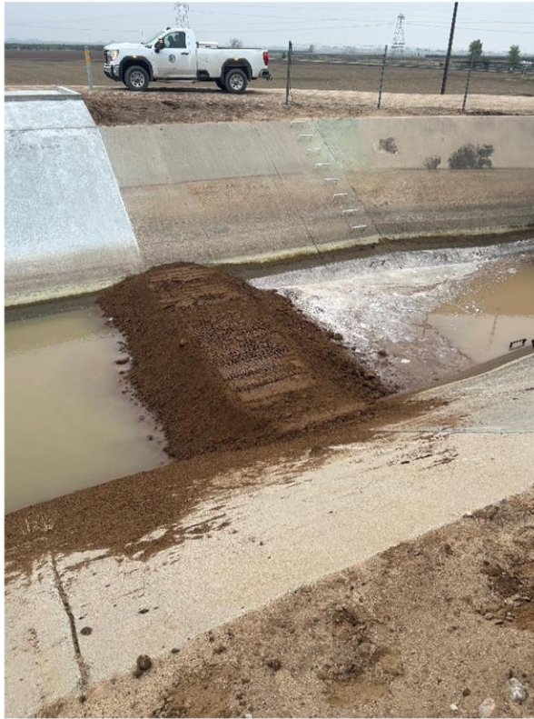
Placed Berm at the Start of North Canal for Winter Maintenance
