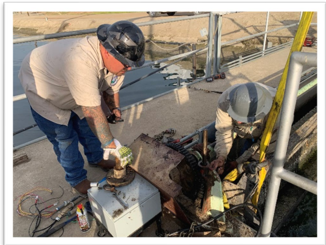
Made Repairs to Check Gate 461
