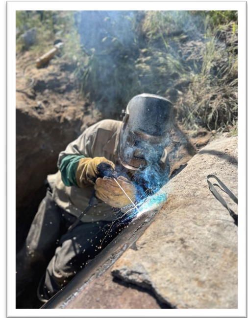
Welded a Patch on a 24-inch N1 Lateral Pipeline
