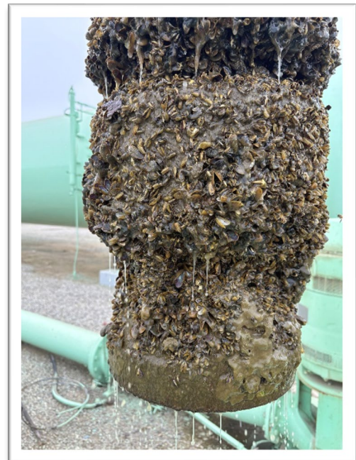
Removal of Vertical Pump at N55-P1 Showing Dead Mussels from Treatment
