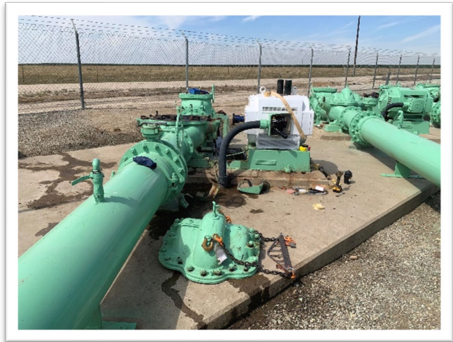
Replaced 10 CFS Rotating Element at Pump Plant N55-P2 Unit#4
