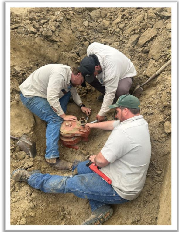
Repaired SC-F Isolation Valve
