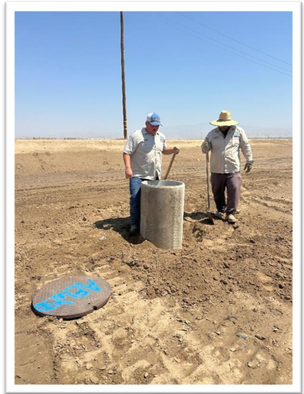
Installed Concrete Rings on Air Vents at North Canal Spreading Works
