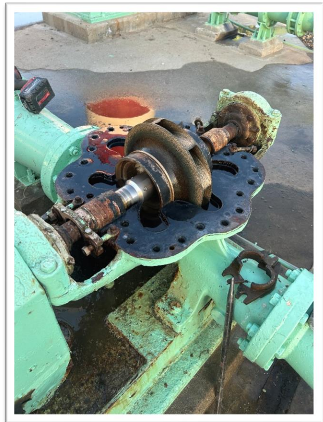
Inspected Pump Plant N55-P8 Pumps and Replaced Packing
