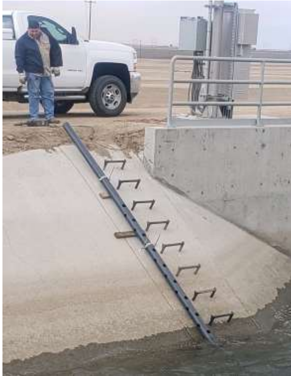
Real Time Water Quality Monitoring Device Installation Underway
