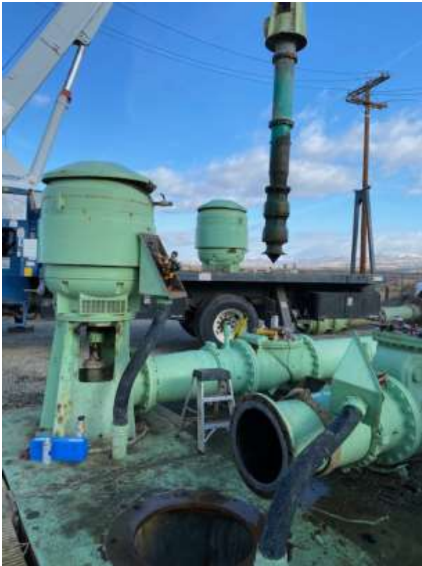
Removing Pumps for Base Plate Modification in Preparation for New Pump Bowls
